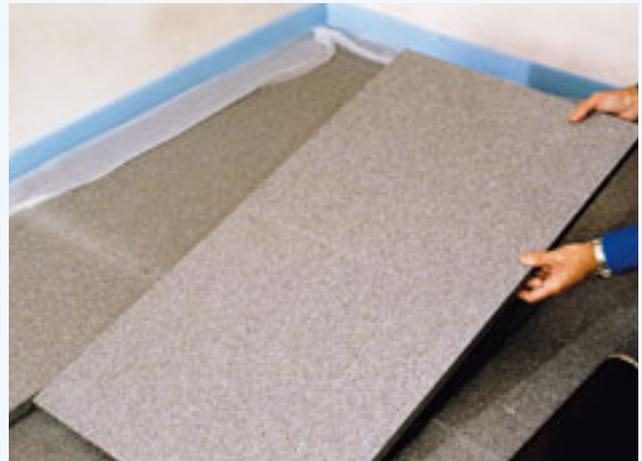
Installation of a Neopor® impact-sound insulating panel.
