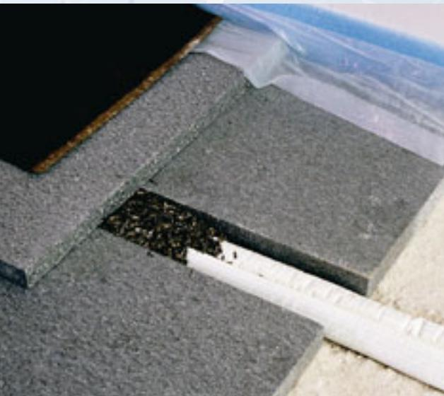
Panels made of Neopor® as leveling layer for pipes laid on the floor
